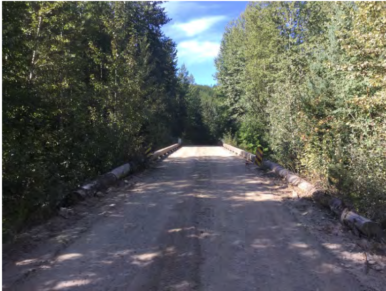
Approach from Right Bank when facing downstream
