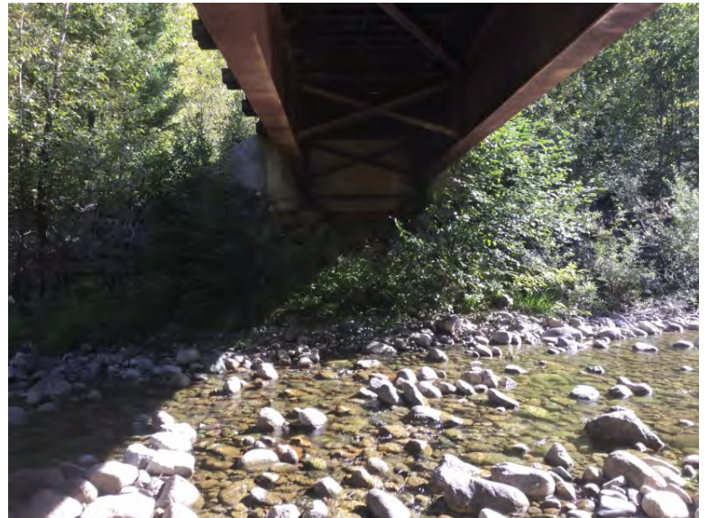
Right Bank Abutment when facing downstream
