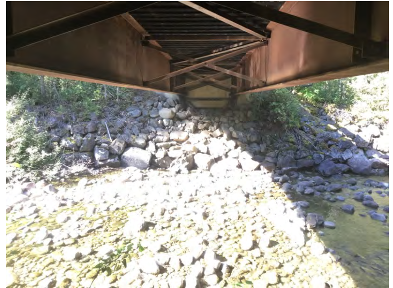
Left Bank Abutment when facing downstream
